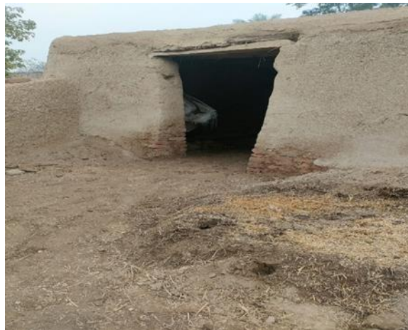
Kitchen from outside
