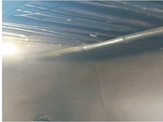
Figure 17 : Roof of Kitchen
