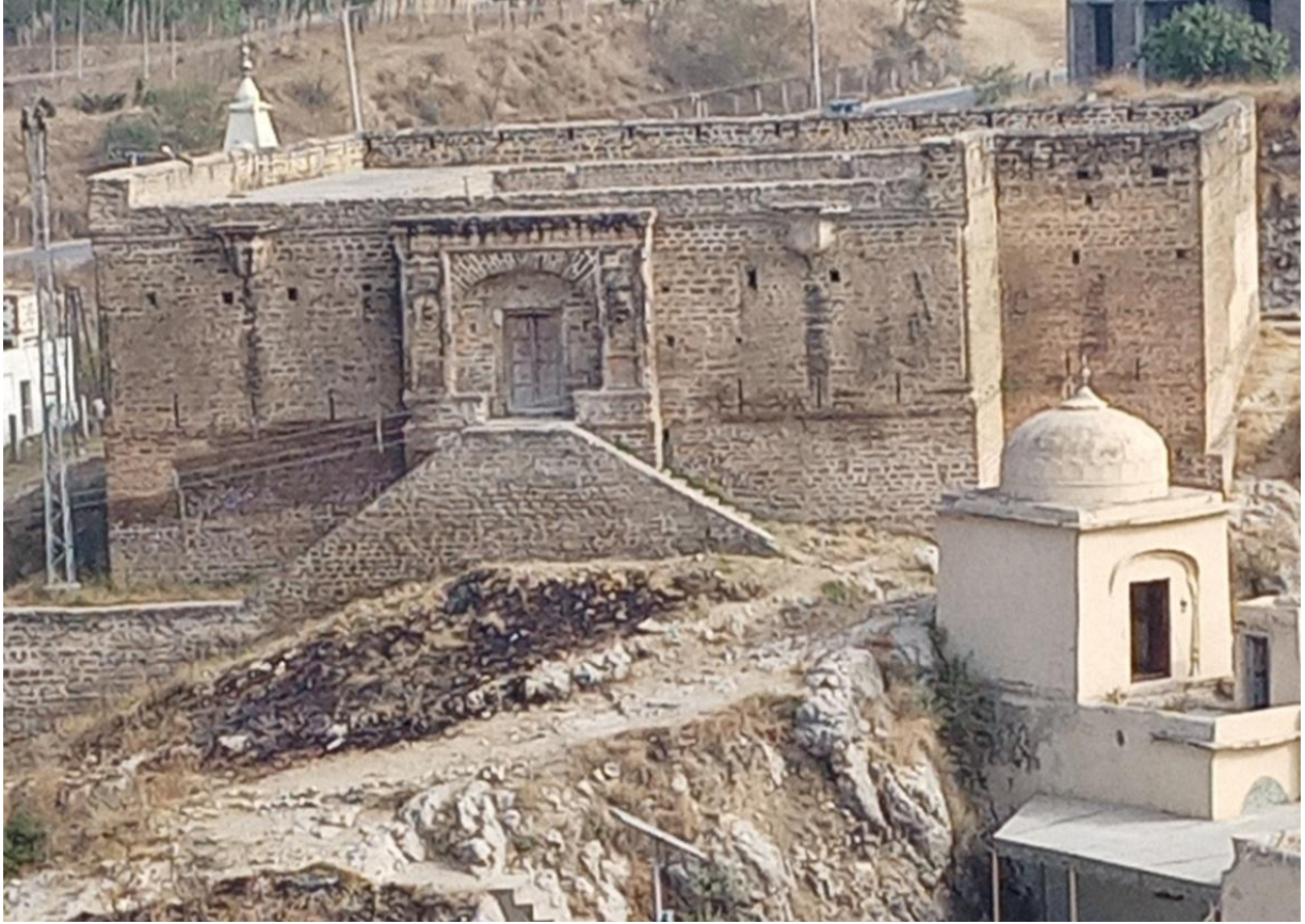
FIGURE 38 POLICE STATION OF KATAS RAJ (BY RESEARCHER)
