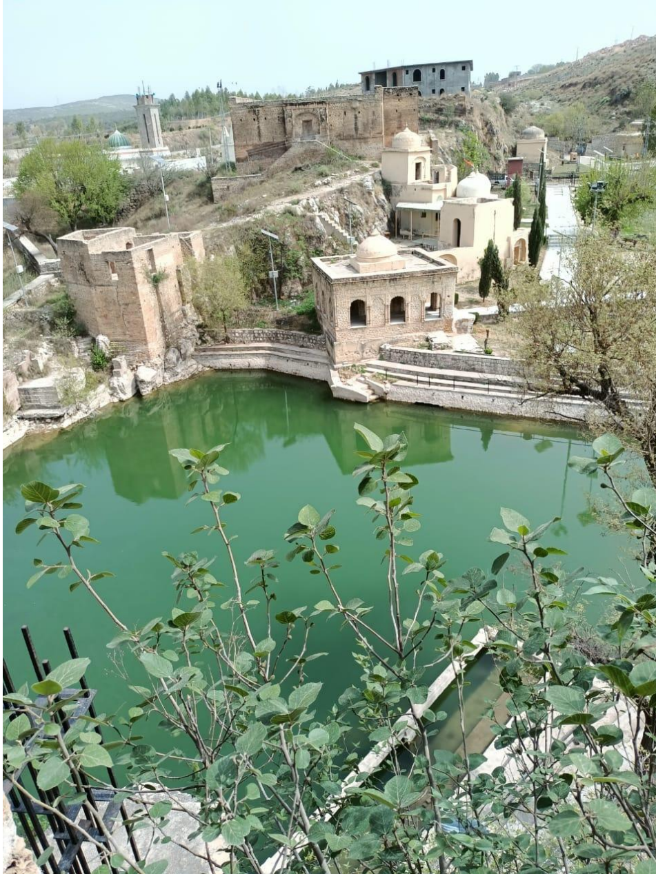
FIGURE 12 A VIEW OF KATAS RAJ TEMPLE COMPLEX (BY RESEARCHER)
