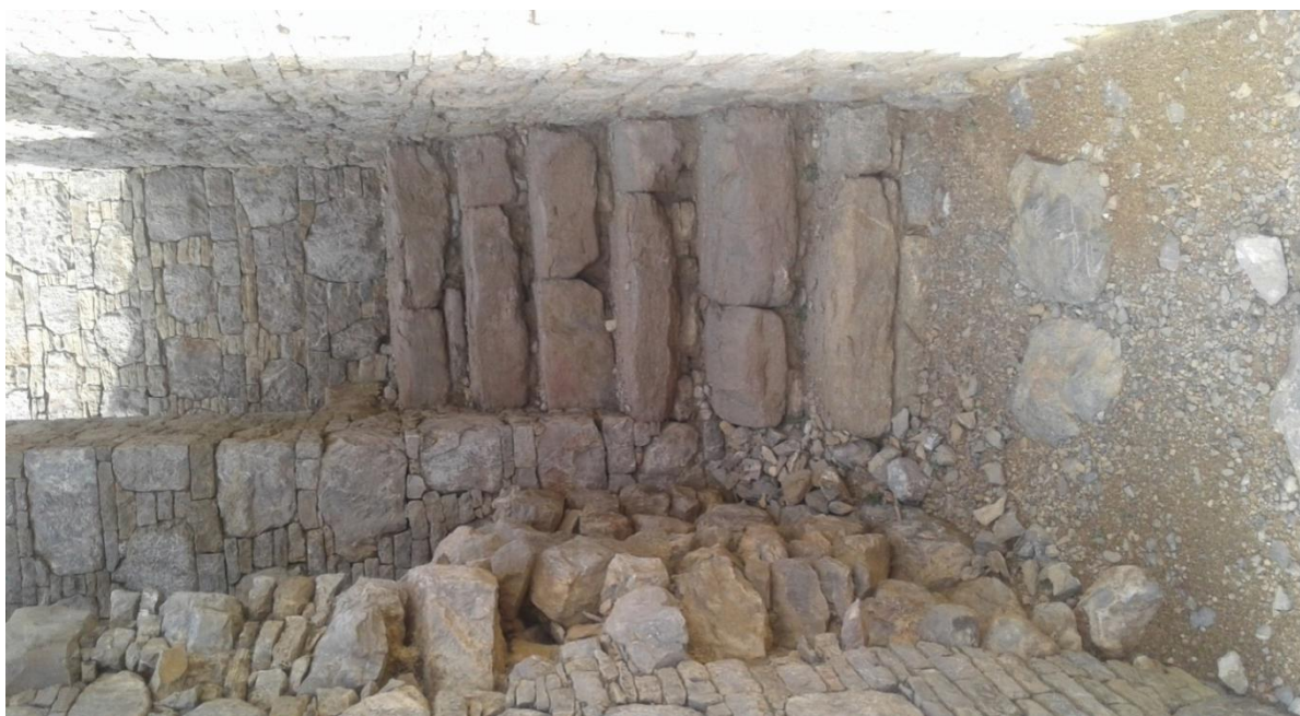
Figure 46: Stairway (Next to the Chamber 8)
