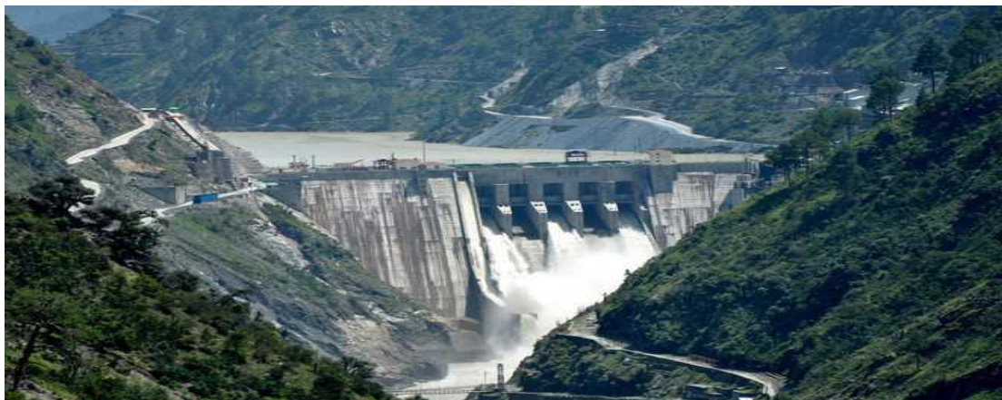
Fig. 3. 5: A view of Baglihar Hydropower Project
