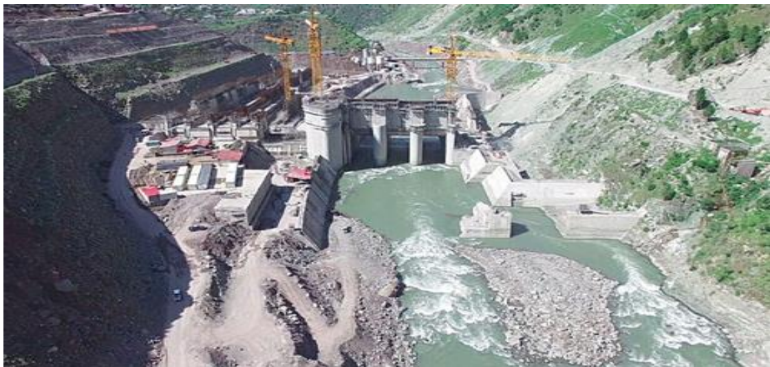
Fig. 3.6: Work on Kishanganga Dam in Progress
